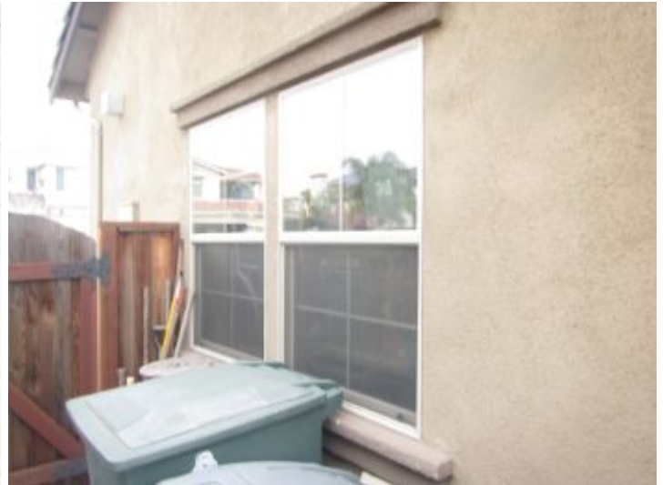
Window at garage
