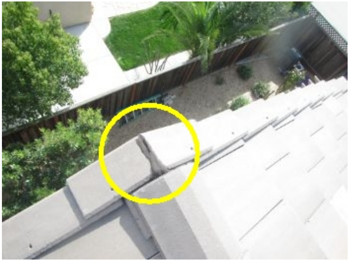
Recommend sealing this edge
